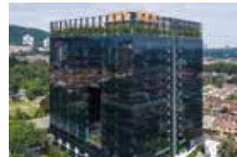
Menara Ken TTDI Sustainable Development
